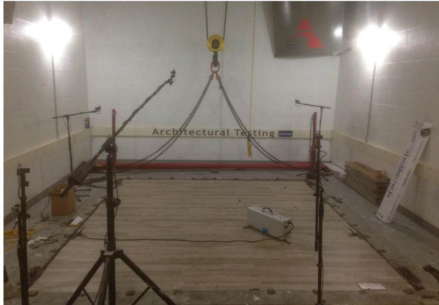
Source Room View of Test Specimen Installation
