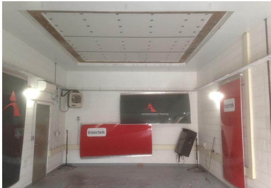
Receive Room View of Test Specimen Installation
